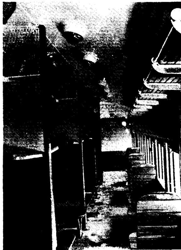
An interior view of the HAL integral coach showing the seats, berths, luggage rack, lights, and fans.
