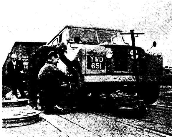
Duthane rail tyres being fitted to a Land Rover for testing.
