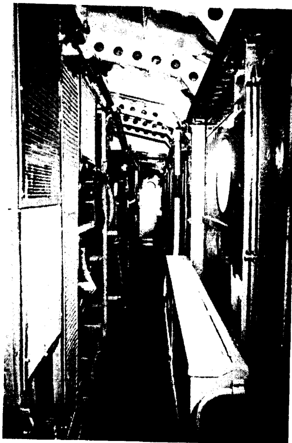
Fig. 19. Inside view of the body in a corridor. The wire netting protects electrical equipment on the left, a quarter of battery set on the right. Looking at the ceiling allows to see the junction between roof and face and their flanges.
