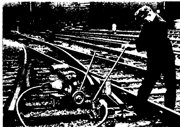
Above: DRILLING a rail ( 1\frac{1}{4} " hole in under two minutes). The under-rail fitting enables the drilling of tracks in use, without impeding the traffic.
