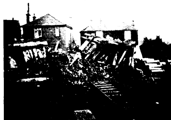
Smashed Earth & Timber Bank to Stop Trains in Marshalling Yard. Friction Buffers have now been installed without any damage to wagons or stops.
