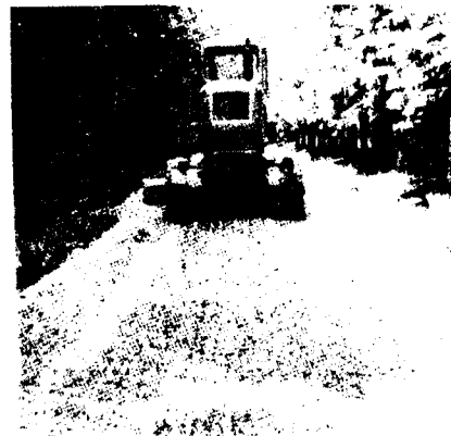
14. Roughening of a sand wearing course with a toothed grader blade during continuous maintenance work
