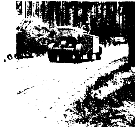
14. Roughening of a sand wearing course with a toothed grader blade during continuous maintenance work
