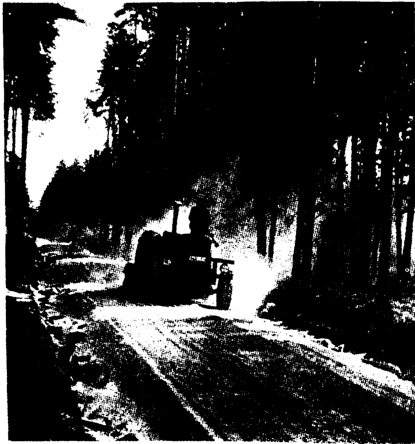
7 7. Mixing quicklime into heavy clay soil
