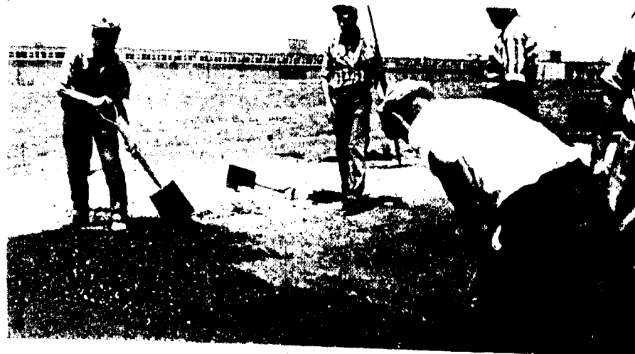
Workers form construction joint. Paper is unrolled over end of roll of welded-wire fabric, which has been secured to pavement with cartridge-fired fastener, and will be covered over with feathered-out hot mix. Normal traffic will use surface, but when construction is resumed paper will be rolled back, stripping away the asphalt and exposing the fabric, ready for lapping with next roll. Below, final step in overlay construction—thorough compaction by rollers
