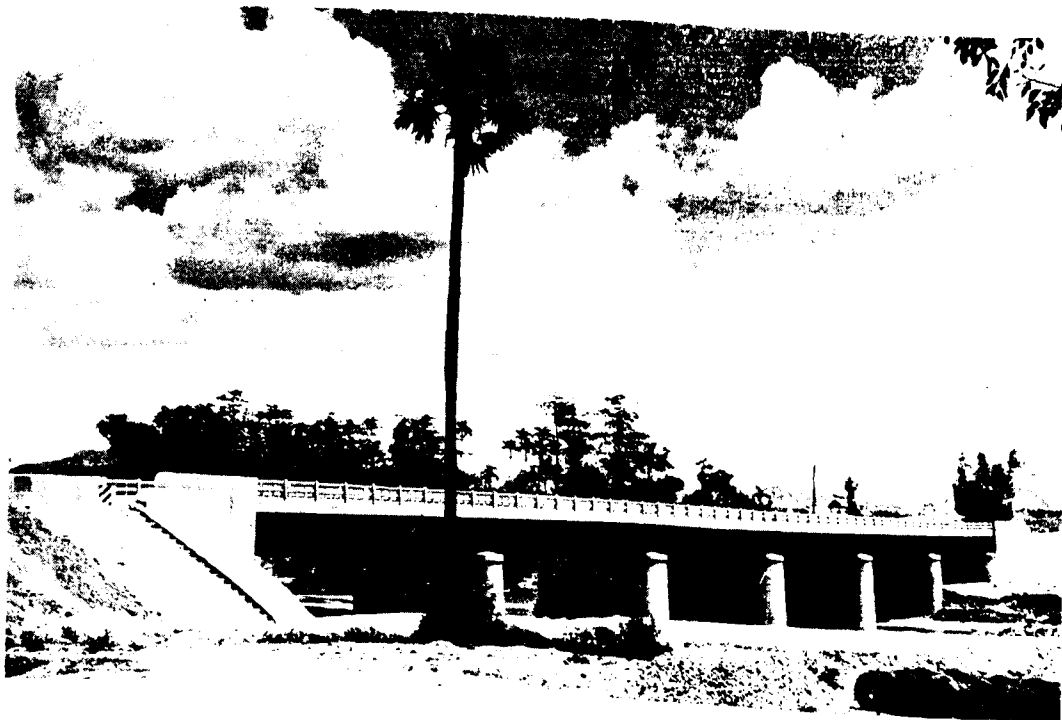
Showing a view of the new bridge from the downstream side
