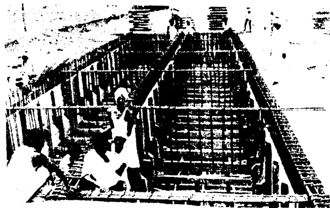
Photo 3. Showing the centering and the reinforcement for the main and cross beams with side shutters for the main beams fixed in position
