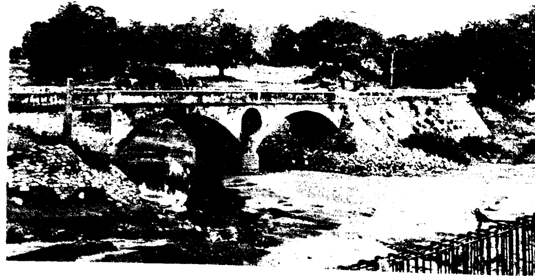
Showing the old arch bridge. Note that the end span on the Bangalore side has been closed and protected by revetment.
