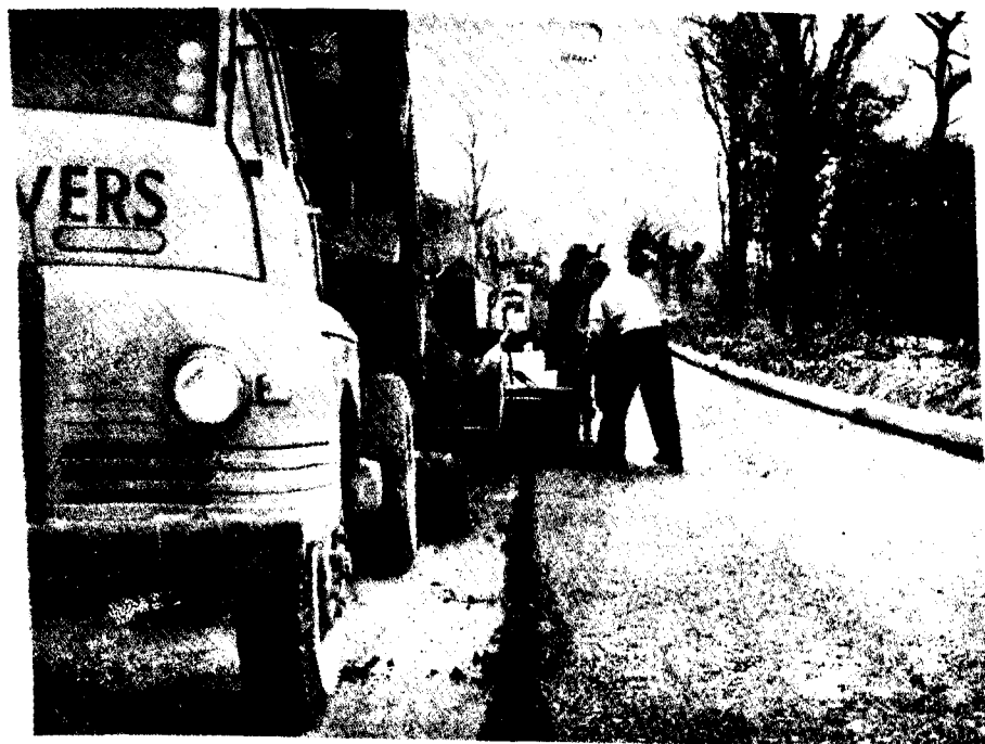
The total thickness of base is built up in 3-in. layers
