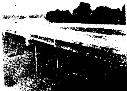
A two-span, prestressed, precast, multiple-beam bridge which was instrumented to provide data. In the concrete construction the Texas Highway Department used sand and gravel in one span and expanded shale in the other.
