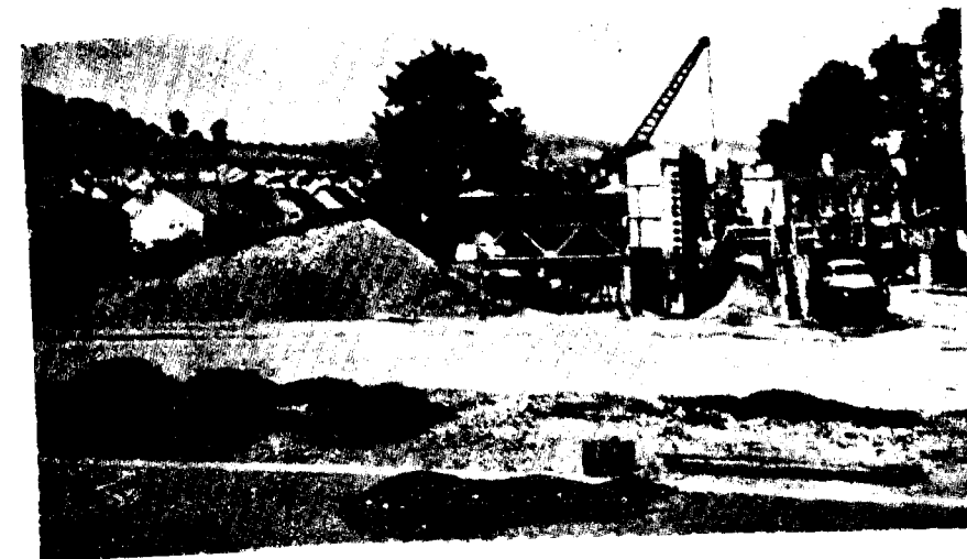
Fig. 4. A batching and mixing plant for lean concrete used in a road base in Glamorganshire. The completed dual carriageway bases can be seen in the foreground
