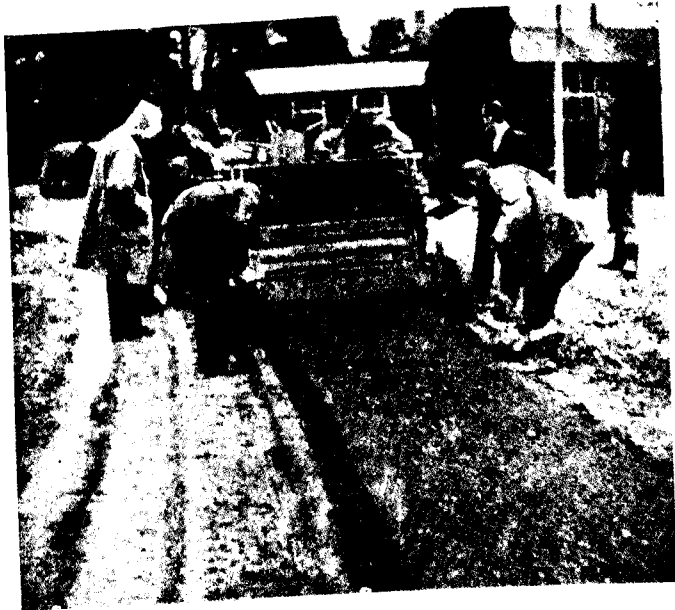
Fig. 9. Constructing a housing estate road in soil-cement using the 4 ft wide Howard single-pass train. Note extent of bulking of processed soil-cement prior to compaction
