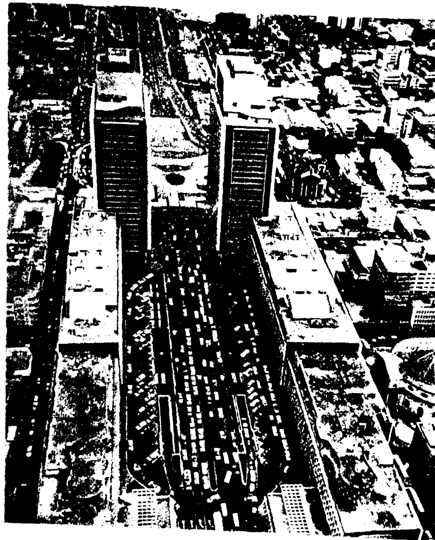
The Centro Simon Bolivar provides for the through flow of traffic between and below office blocks with elevated pedestrian ways and under-ground parking for 1,600 cars
