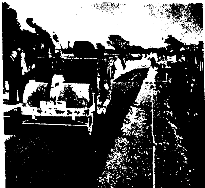
Fig. 6. Compacting a soil-cement road base with an 8-ton smooth wheeled roller. Note white tape laid as a guide to tractor operator of 6 ft Howard single-pass train
