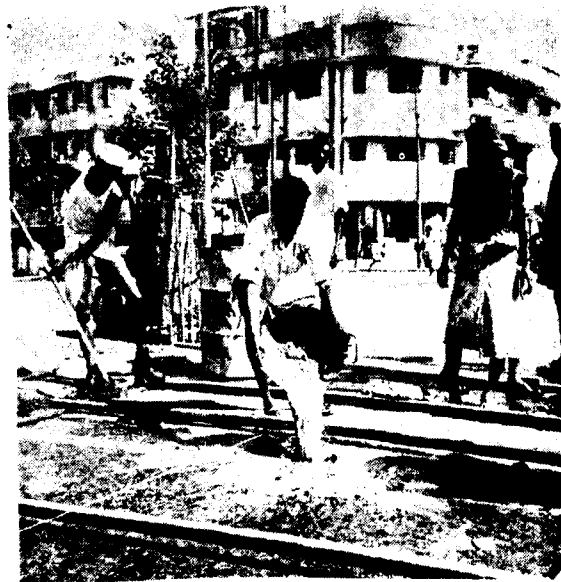
Pouring cement-sand grout (1 : 1 mix) on the treated surface and spreading the same uniformly by a brush, prior to laying the resurfacing
