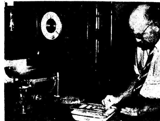
Shape-test of aggregate
