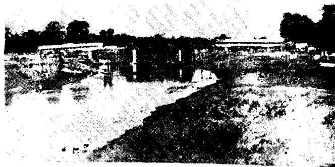
R.C.C. Bridge over Kullong River at Nowgong (Assam) (under construction)
