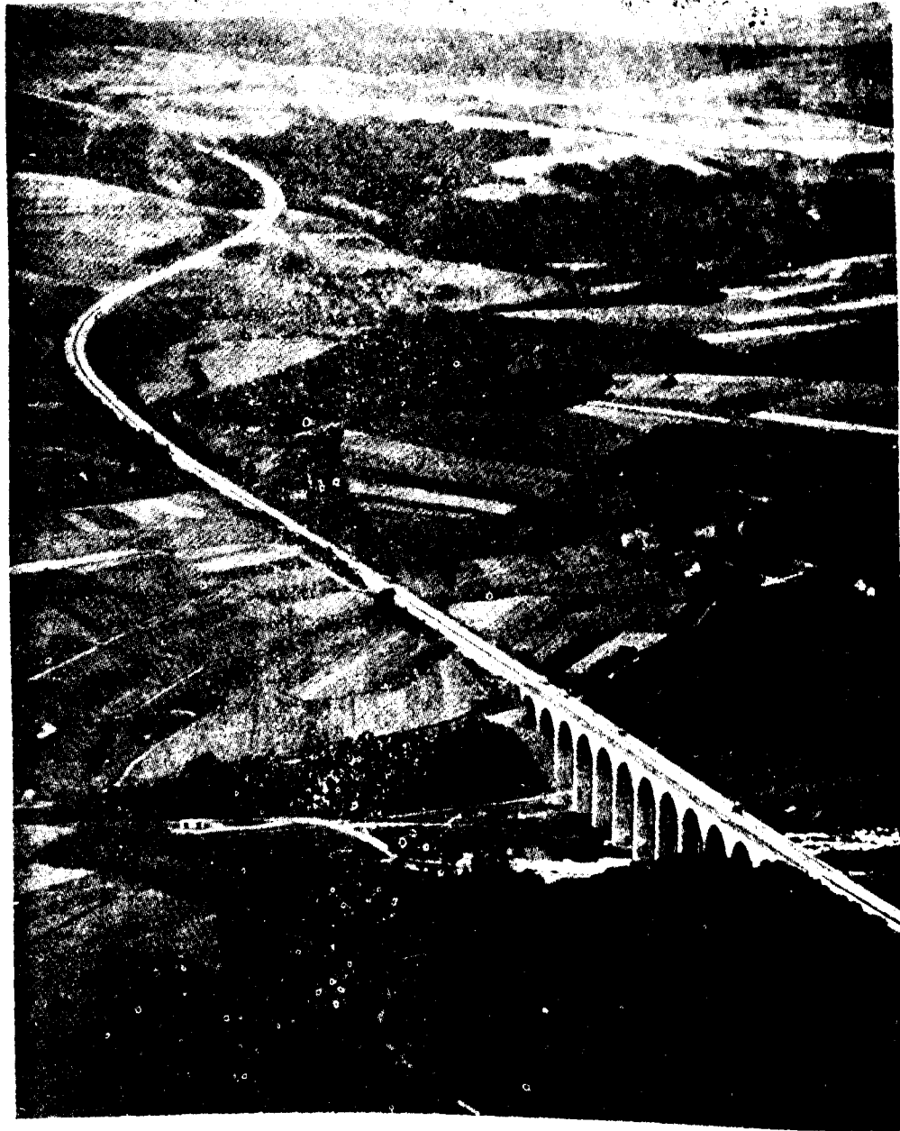
Photo 3. Wiedbachtal bridge along the Cologne—Frankfurt autobahn
