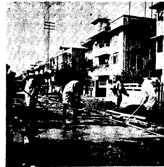
Spreading the diluted acid on the existing concrete surface and brooming the same evenly by a light brush to produce a good effervescence
