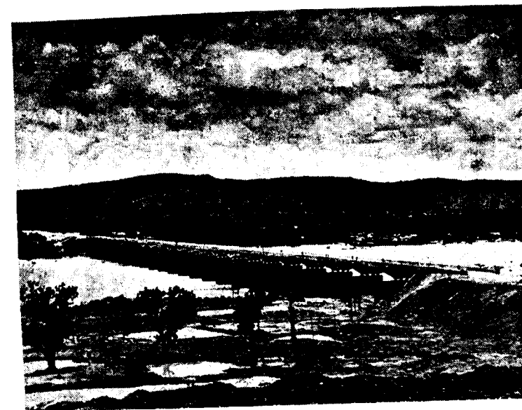
Mahanadi bridge at Sambalpur
