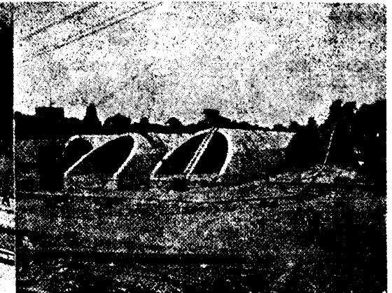
Ross By-pass — Wye Flood Plain. Four of the flood arches under construction over which the embankment will be built up
