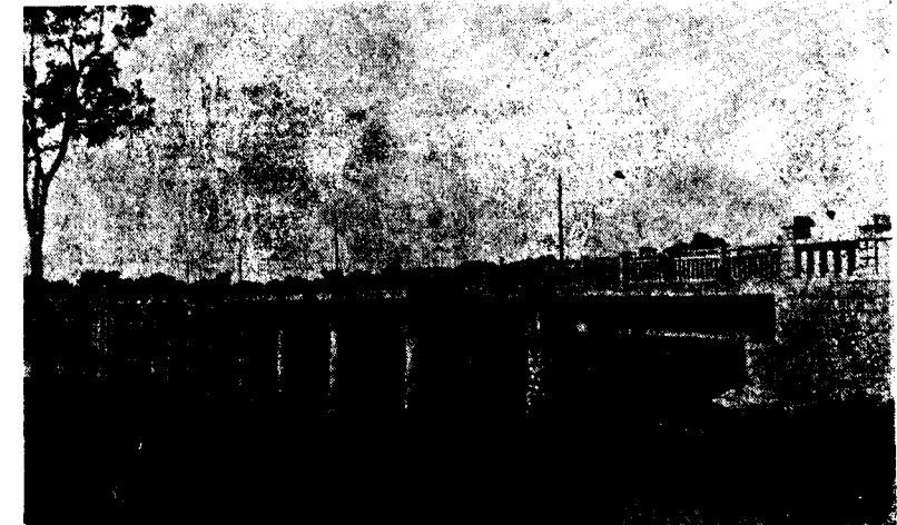
Bridge across the river Cauvery near Bannur
