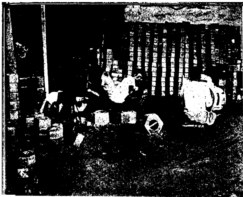
Fig. 3—After the metal has cooled and solidified, the moulding boxes are opened and the rough cast weights are taken out. It is necessary to chip off protruding edges and surplus metal from the castings before they are taken up for finishing. The picture shows fitters chipping off the excess metal.
