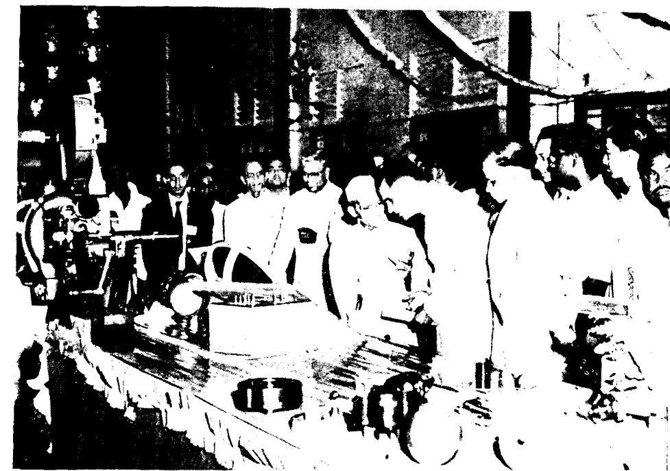
Shri Lal Bahadur Shastri and Shri Manohar Malaviya are seen in the workshop. They are inspecting the machine in the workshop. The machine is kept in use in the Industrial Estate.
