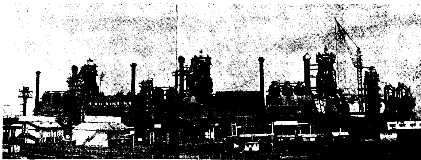
Blast Furnace Plant at Bhilai
