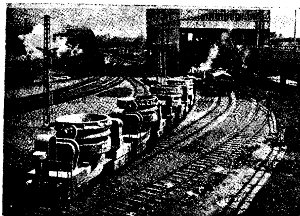
Slag transfer cars with automatic pot locking
