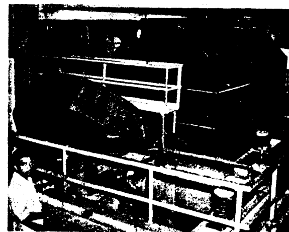
Interior of Coal Washery Plant at Durgapur Steelworks.
