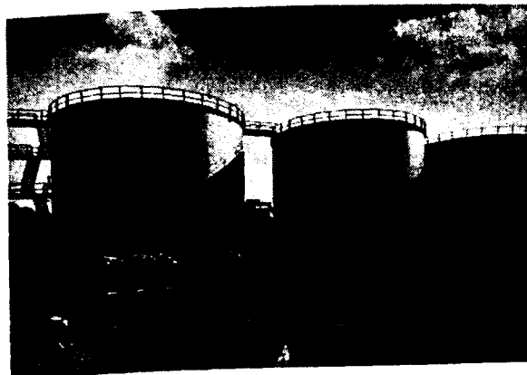
These 600,000 gallon storage and the walkways and stairways have been treated with Plus Gas Formula 'E' External Metal Treatment prior to the normal painting process. This photograph shows the smooth surface achieved by this process which was applied over a heavily scaled surface.
