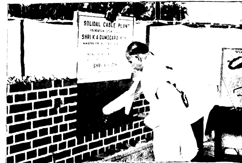
Solidal Project : Mr. K. A. Damodara Menon, Industries Minister, laying the foundation stone
