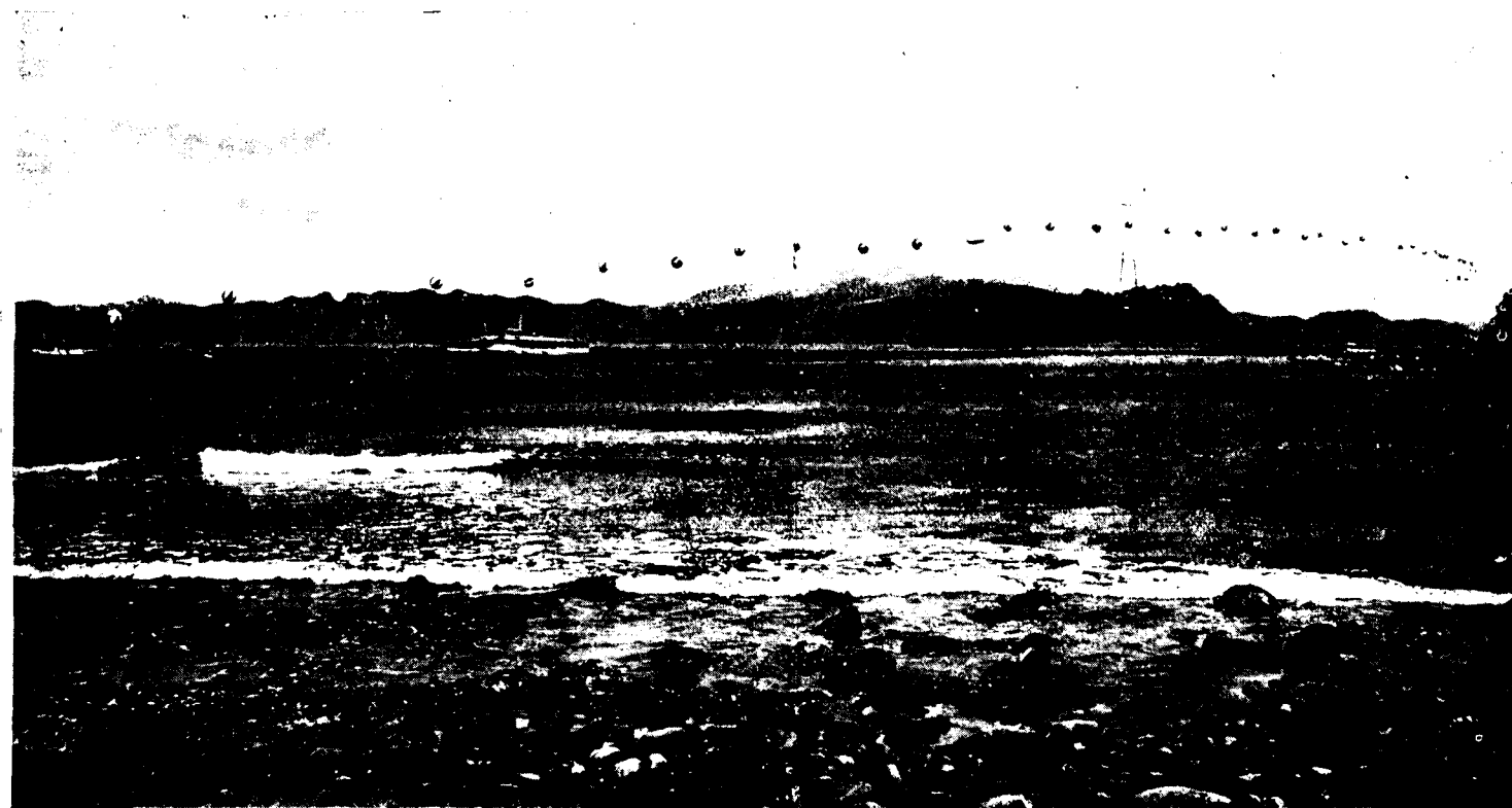
Across Naruto straits : Seventy-seven multi-coloured balloons were used on a stringing operation
