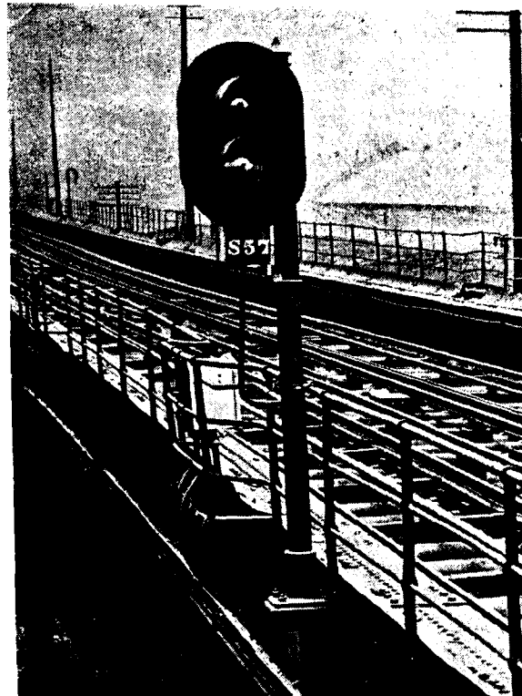
First colour light signals installed in United Kingdom. A two aspect signal on the Liverpool Overhead Railway.
