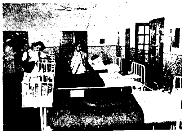
Interior view of the new Maternity Block in the Railway Hospital at Khargpur.
