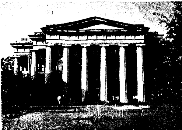
An exterior view of the Railway Hospital at Garden Reach. This majestic building was once the residence of the Railway's General Manager.
