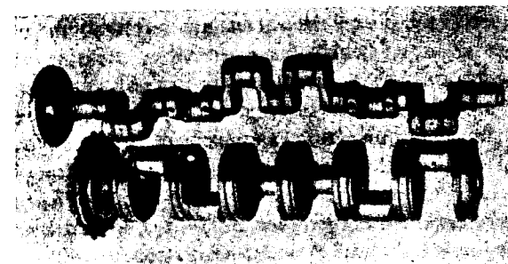
Fig. 3. Conventional and disc webbed crankshafts illustrated to show the increased strength and rigidity of the latter.
