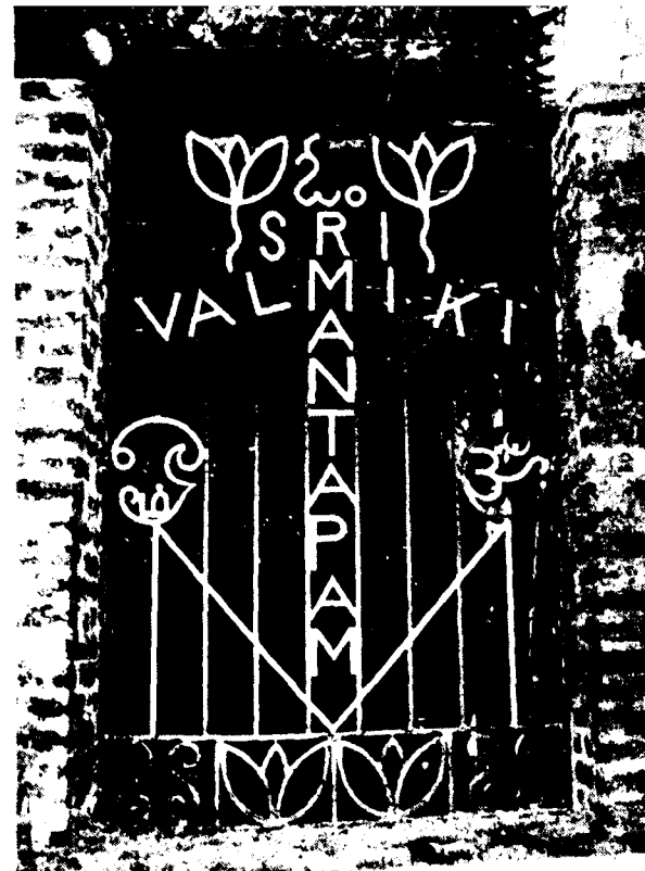
One of the eight artistic iron grillwindows fitted in the walls of Sri Valmiki Mantapam (Sri Thyagaraja Shrine Thiruvaiyaru, Tanjore Dt.)
