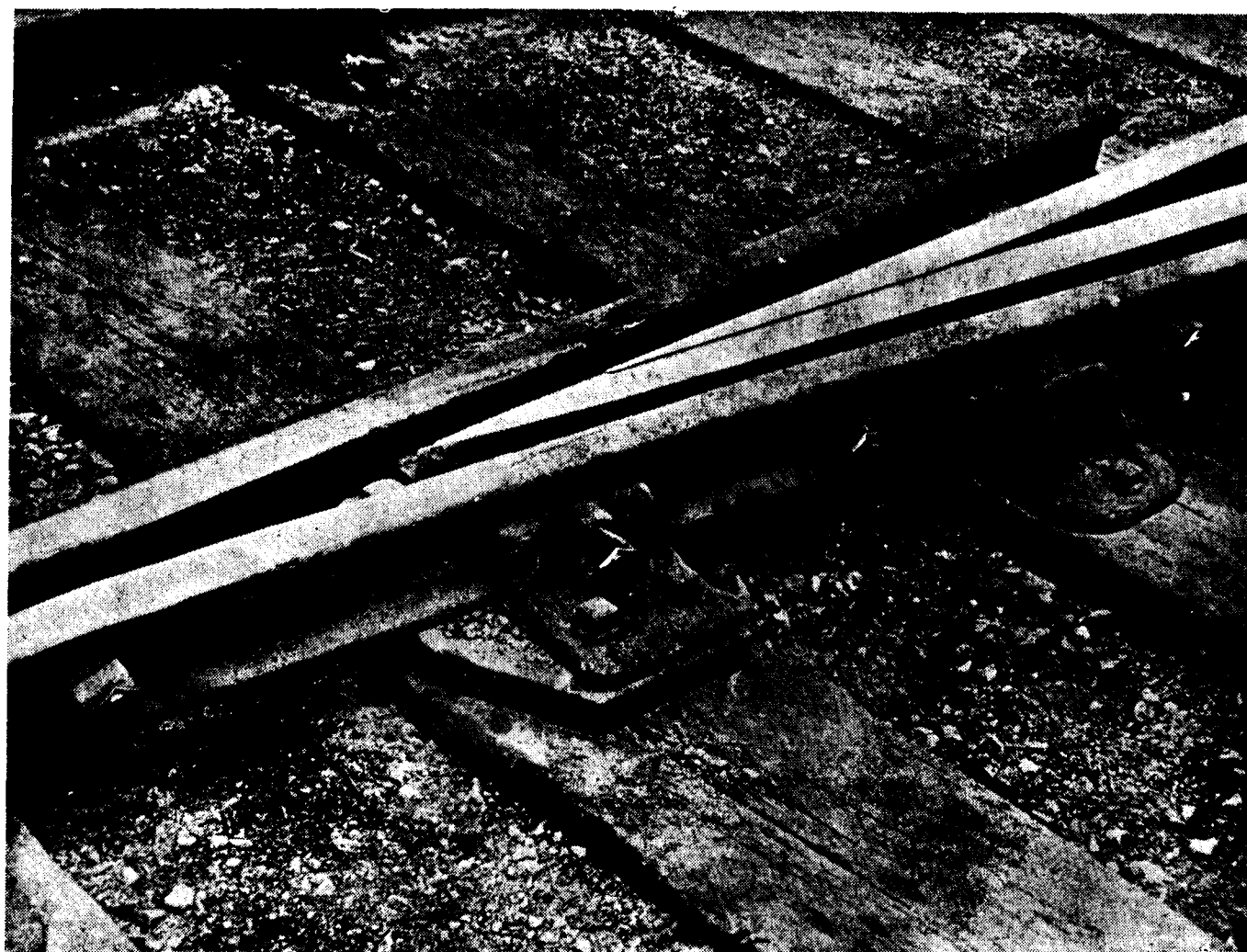
Photograph by courtesy: British Railways (Western Region) West Ealing "Palnut" Safety Lock Washers Crossing Bolts.
