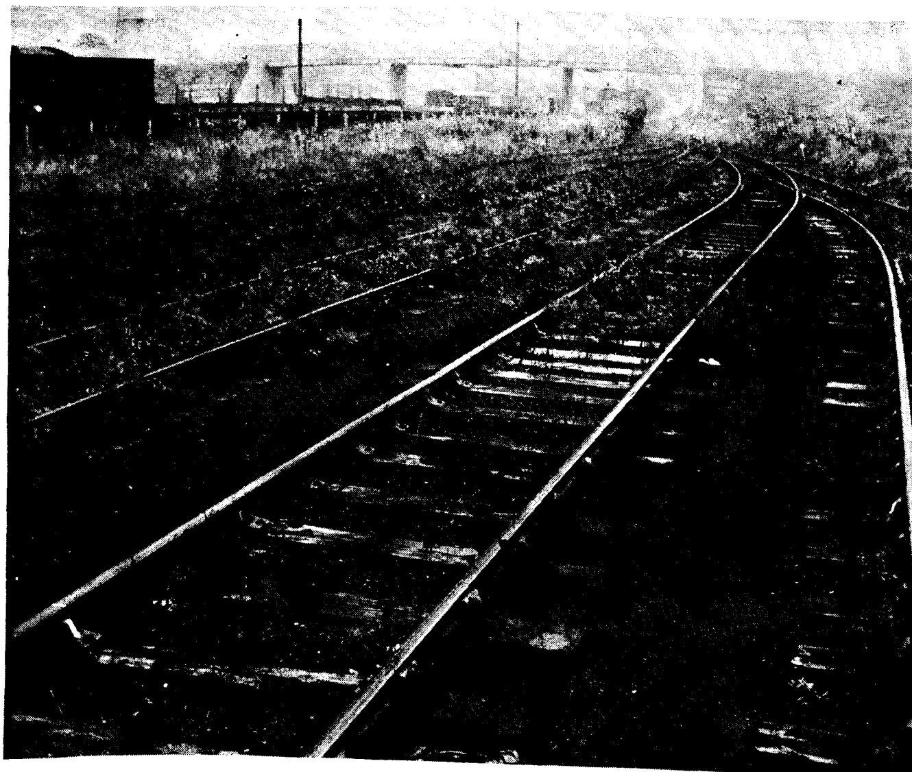
Photograph by courtesy: Fisons Pest Control Ltd., U.K. Weed infested railway tracks—Foreground treated with Simazin.
