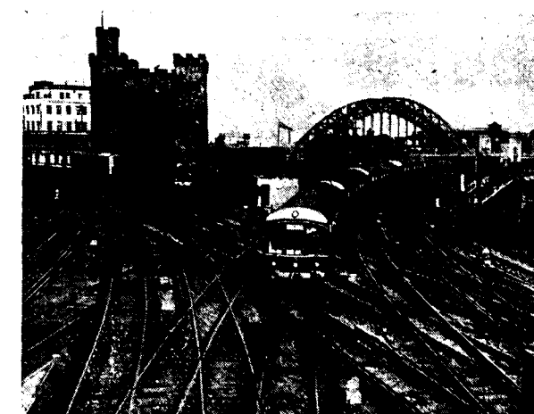
Typical British Railways 4-car multiple unit train at Newcastle. These trains feature B.U.T. 150 h.p. horizontal diesels, transmission and control equipment and can be operated in multiples up to twelve cars.
