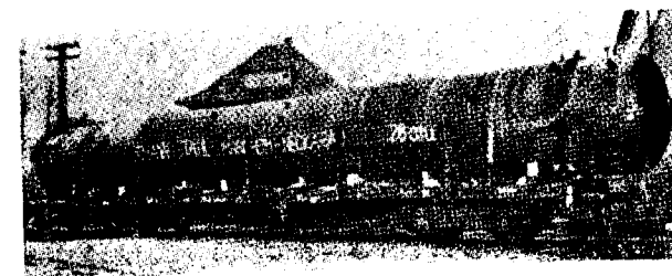
Fig. 26. CO-Washer welded with low-hydrogenelectrodes. (Photo : Johann Stahl, Mannheim-Neckarau).
