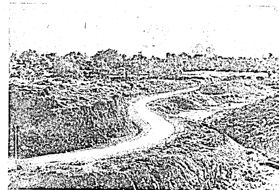
A completed section of a National Highway
