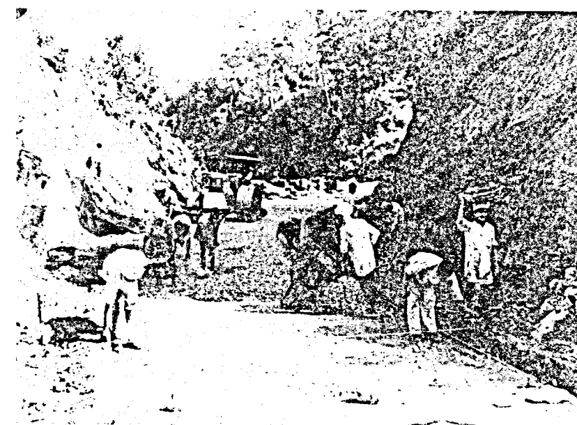
A road under construction
