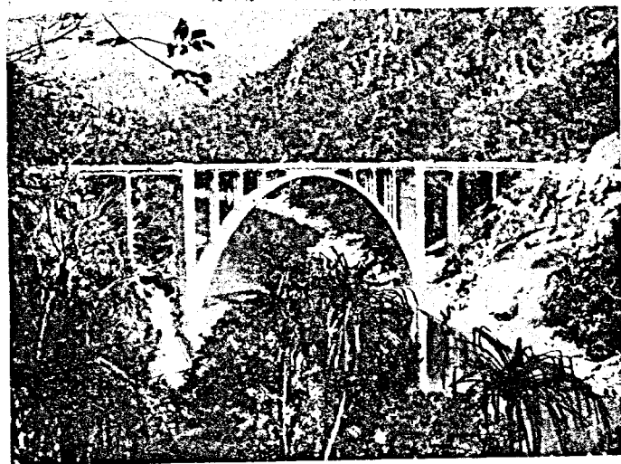
An Indian concrete arch bridge of unusually high rise. The Coronation Bridge over the Teesta in West Bengal has a span of 276 feet and a rise of 132 feet. The arch is of hollow box section and was built in 1941 by the Public Works Department of West Bengal.
