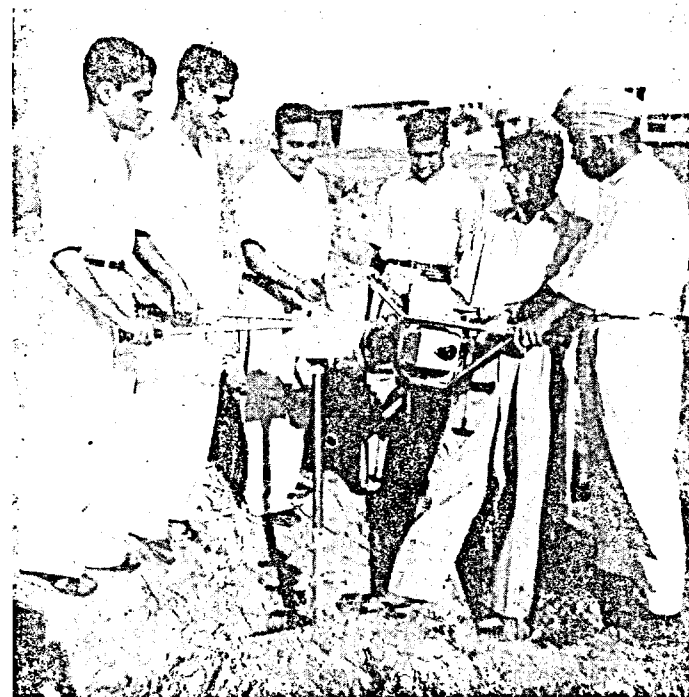
Picture shows the post-graduate students trying out the Power Auger at the new swimming pool tank site
