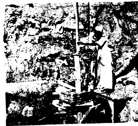
Photo 3. Plate Bearing Test Assembly in position
