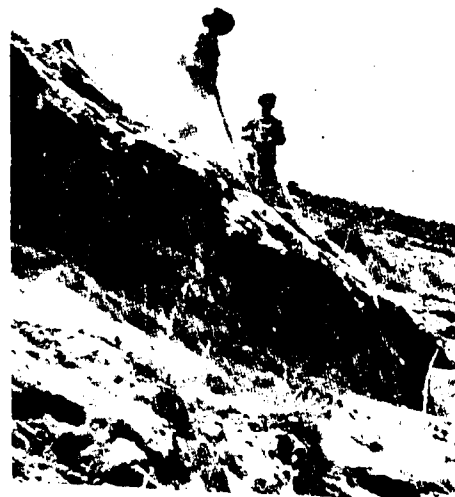
Jerusalem-Hartuv road. Typical view of terrain prior to earthworks
