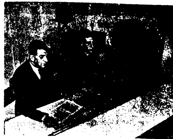
Mr. R. Hills (left) chief executive of the A.R.A. at the supersonic tunnel control panel.
