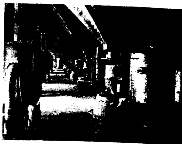
Upper level of gas generators with fuel bunkers, semi-automatic feeder and boiler.
