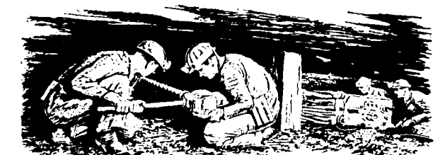
Coal released from its primordial prison by drilling and then applying explosives.
