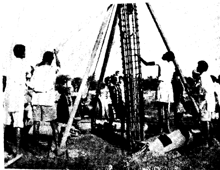
The above view shows work in progress on the construction of 19" diameter Piles For DHAMDACHA Bridge in Navsari Dangs Division for Bombay P.W.D.
