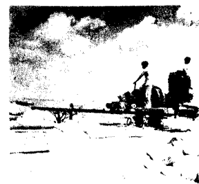
Photo 1. 15 H.P. diesel winch mounted on trolley for extraction of piles
