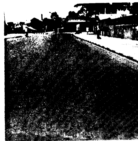
Photo 1. Bus stop on Whannels Road laid on water-bound macadam in February 1957
