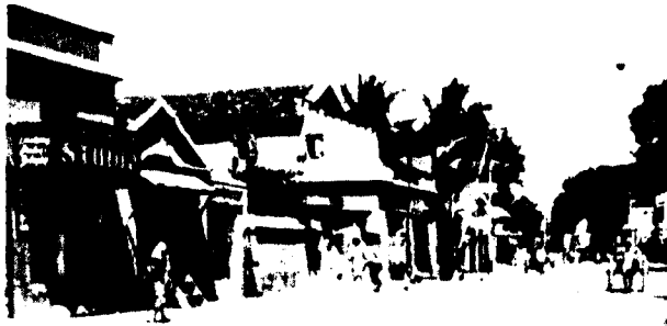
Photo 4. Egmore High Road surfaced in July 1958
