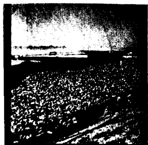
Photo 9. Another view of boulder apron partially submerged under water. In front is the subsidiary channel successfully blocked
