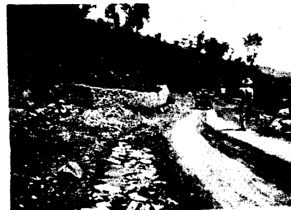
Photo 12. Bare hills, boulder sausages and a new diversion opened for traffic
