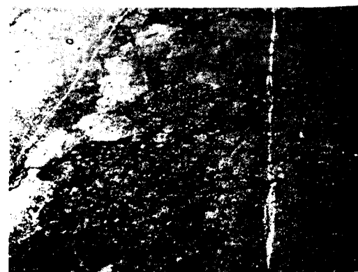
Photo 3. Surface cracks in M 31/4, result- ing from inade- quate thickness of pavement
