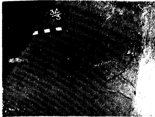
Photo 16. The same hair cracks of Photo 15 marked with a pencil for clear presentation
