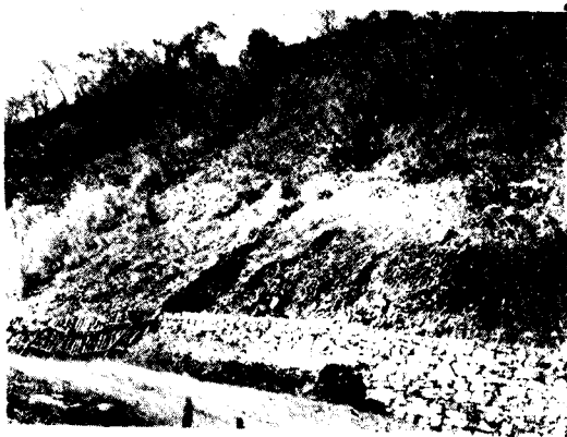
Photo 14. Boulder sausage and jungle wood palisading
