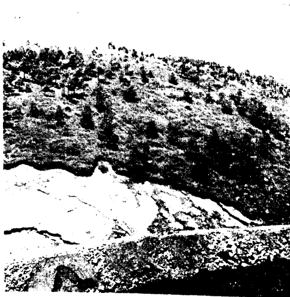
Photo 9. Face of secondary slips
