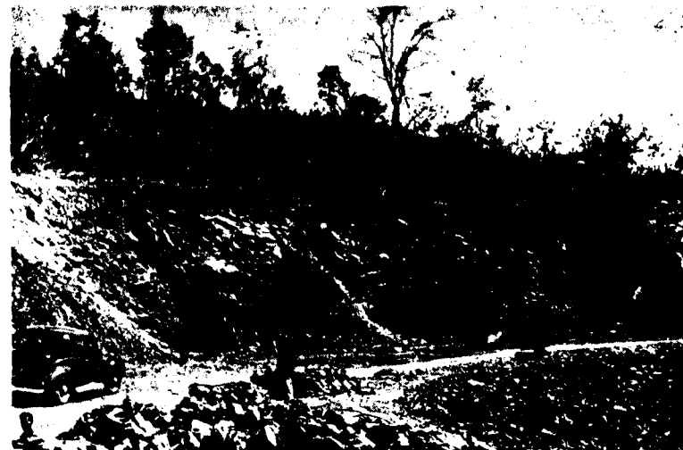
Photo 7. Landslides in bare hills due to disintegration and weathering
