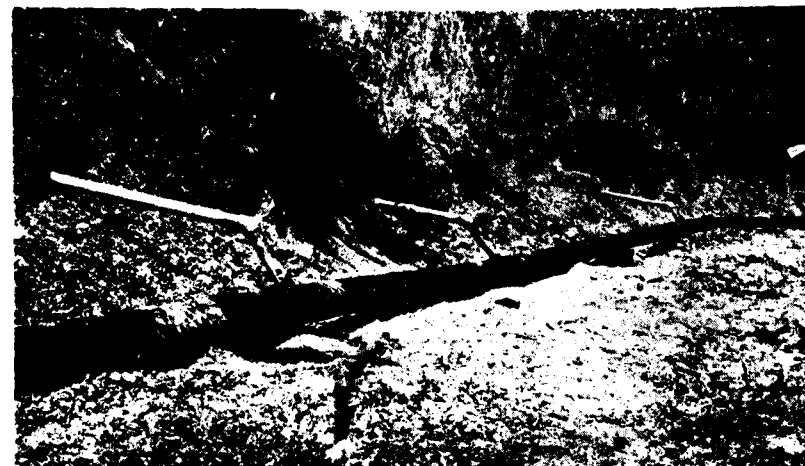
Photo 8. Horizontal drains working to release the hydrostatic pressure
