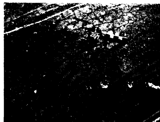
Photo 1. Surface cracks in M 28/7, resulting from inadequate thickness of pavement
