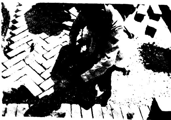
Photo 4. Laying of brick-on- edge in herring- bone bond
