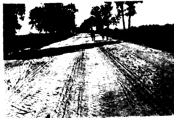
Photo 7. The pave- ment under traffic (note the earth blinding on top)
