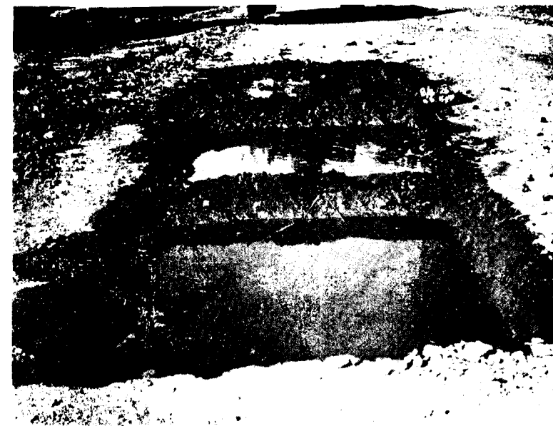
Photo 2. Stepped up pit under soaking for 24 hours at mile 8/7 of Batala-Siri Hargobindpur road
