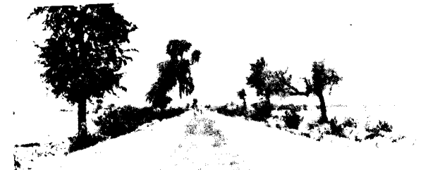
Photo 12. General view of reconstructed portion (mile 7.4) of Batala- Siri Hargobindpur road after a year's traffic
