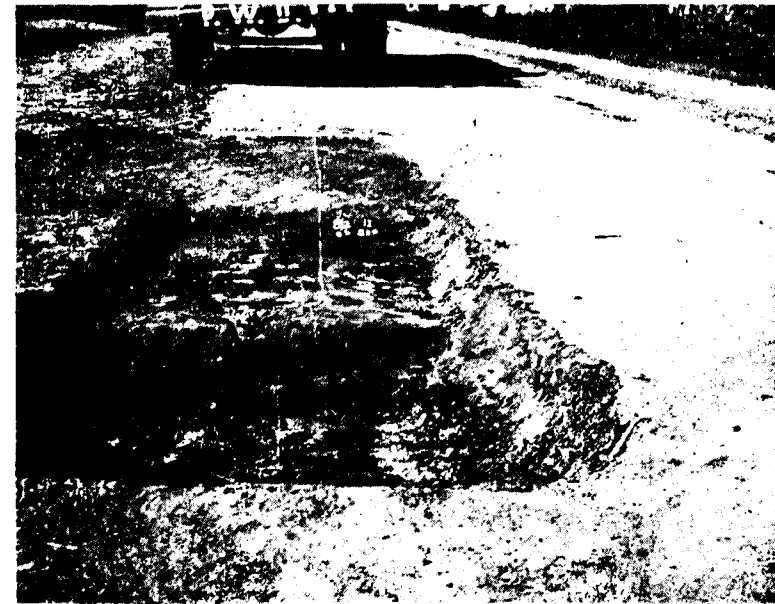
Photo 1. Stepped up pit before soaking at mile 8/2 of Batala-Siri Hargobindpur road
