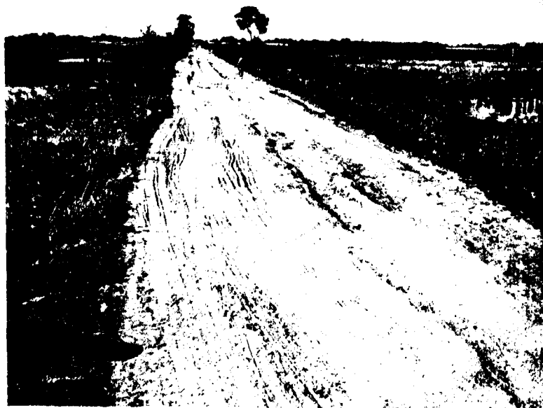
Photo 4. General view of the waterlogged area on both sides at mile 7/8 of Batala-Siri Hargobindpur road
