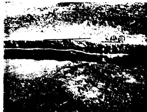
Photo 5. Cross-section of mile 7/8 (failed section) of Batala- Siri Hargobindpur road. The uniform thickness of wearing course and the complete sinking of all the layers may be seen
