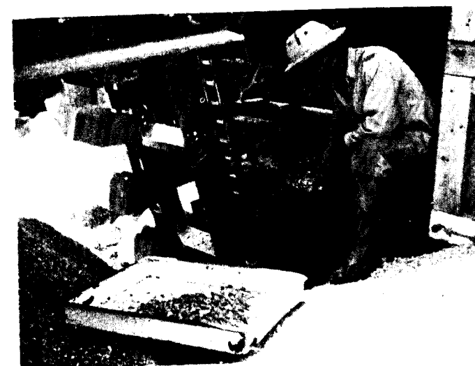
Photo 8. Sampling at cold elevator
