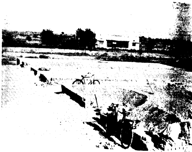
Photo 16. Storage bins of aggregates at the plant site
