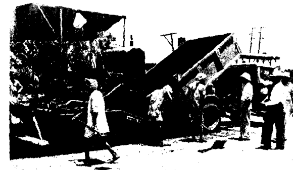
Photo 3. Paver being loaded
