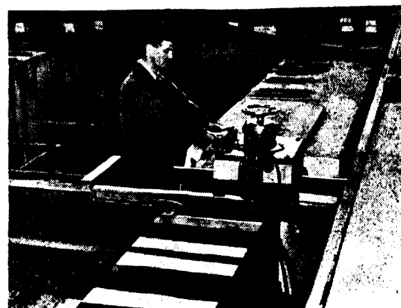
The Illustration shows a "WRIGHT" Model 1.5/2P Self-Contained Motorised Grinding Head, Flange Mounted into a four-wheeled Bogie, running on Rails and in this instance being used for surface-truing of turbine foundations.
