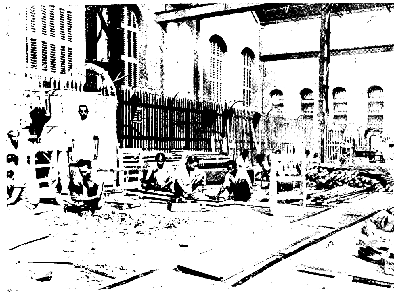
General view of sub-assembly section.
