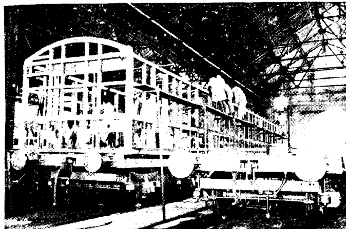
Skeleton Body of the Coach under construction.
