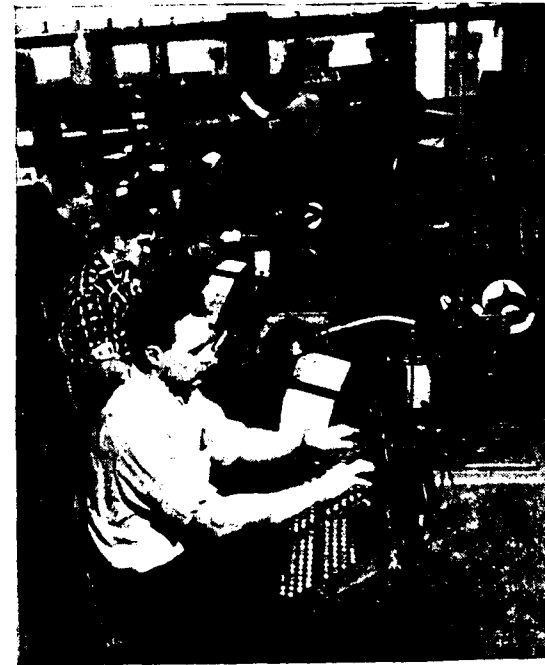
These apprentice students are learning to operate a monotype key-board for the casting of individual type characters.
