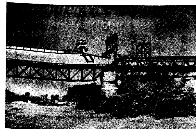
New girders almost completely lowered.
