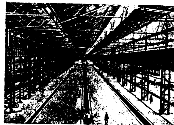
Service Trenches inside Shops.
