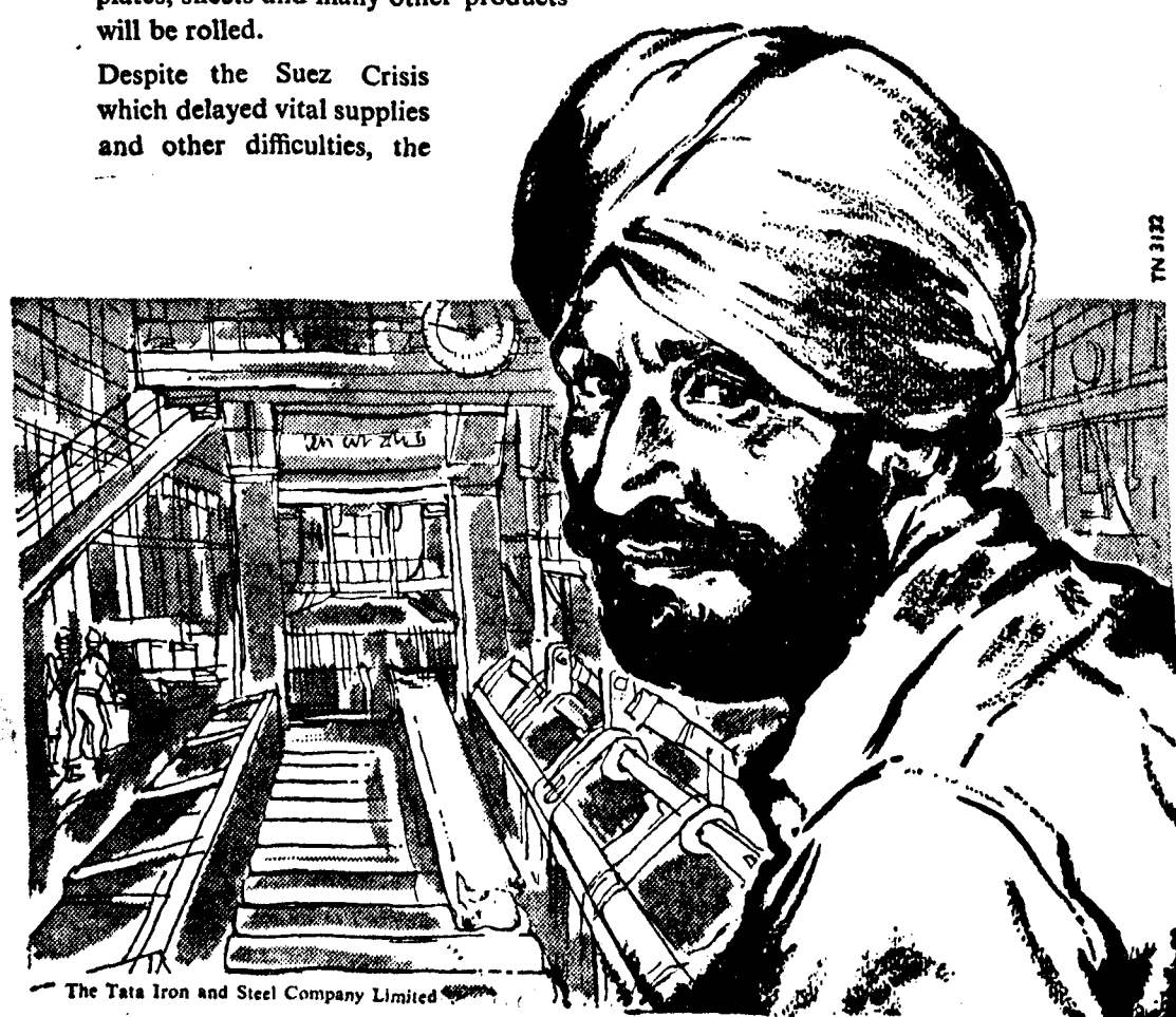
The Tata Iron and Steel Company Limited
