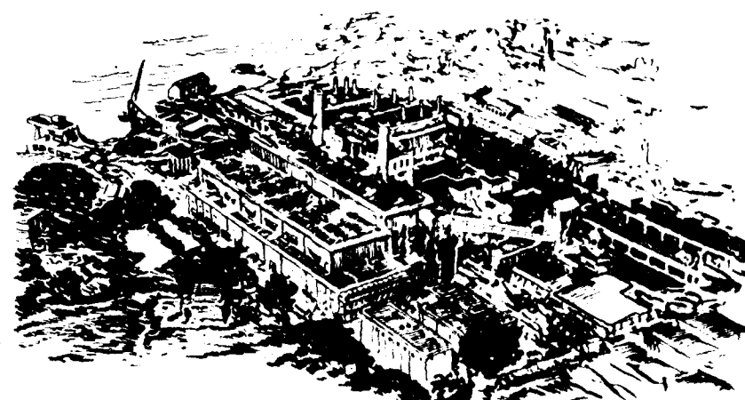
NEW COSSIPORE POWER STATION—CALCUTTA
