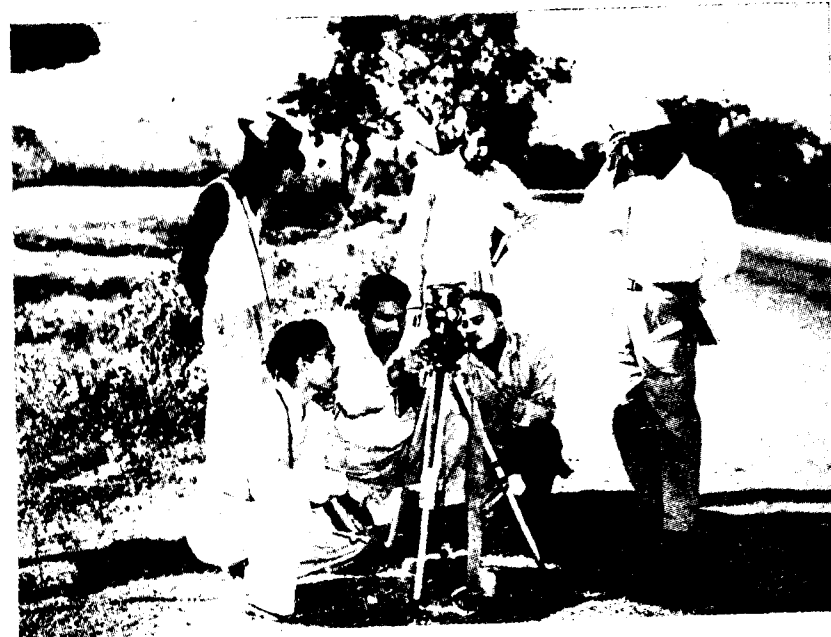
GSI trainees setting up a theodolite instrument to make preliminary surveys for topographic maps.
