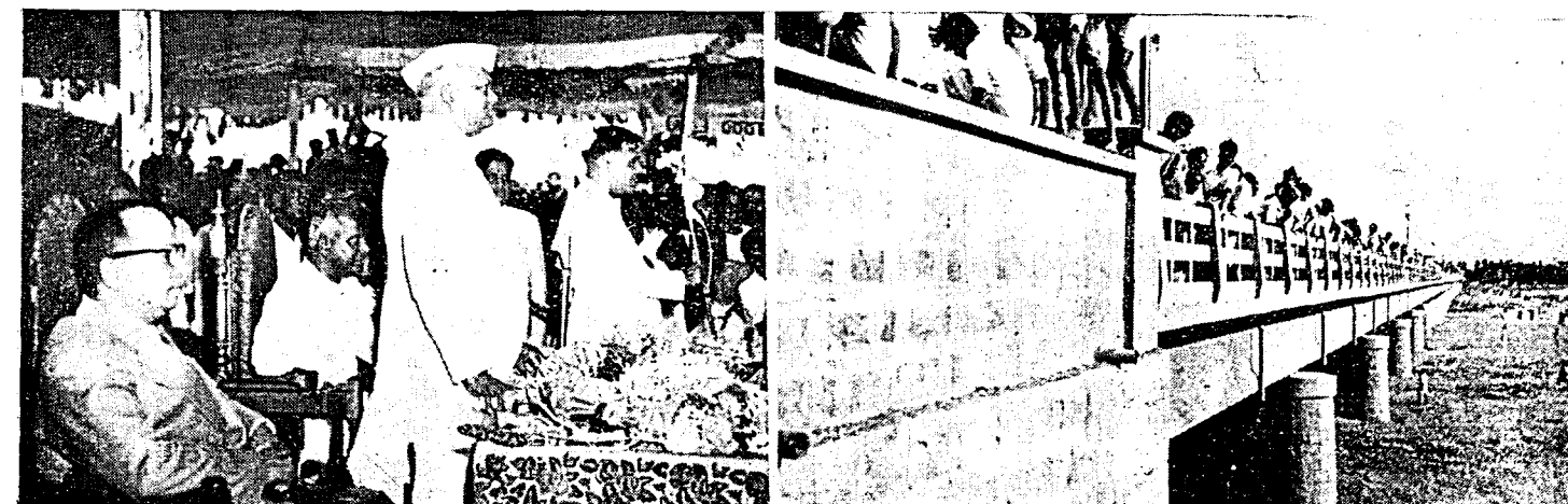
A bridge across the Palar near Ranipet was declared open on 20th July 1959 by Sri Raj Bahadur, Deputy Minister for Transport and Communications, Government of India.
