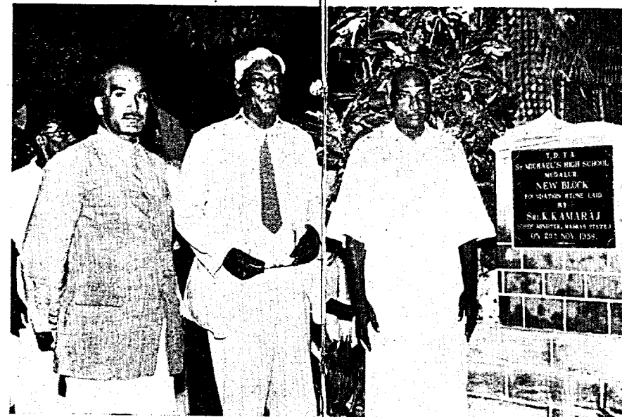
(5) . . . laid the Foundation Stone for new block of school building at Mudaliar . . . .
