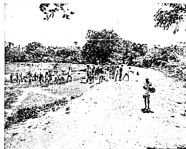
Laying a Road.
