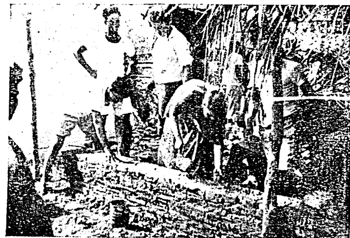
A hut under construction.
