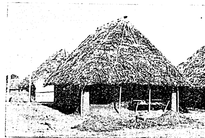
Dwellings under construction.
