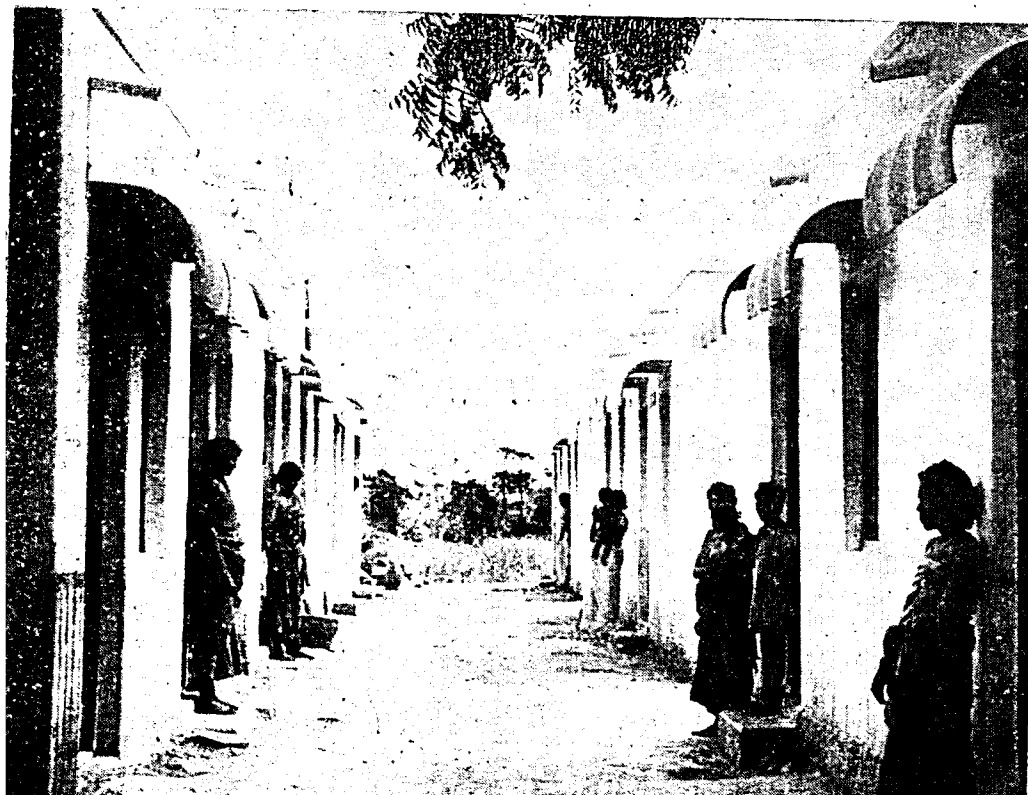
The rebuilt houses.
