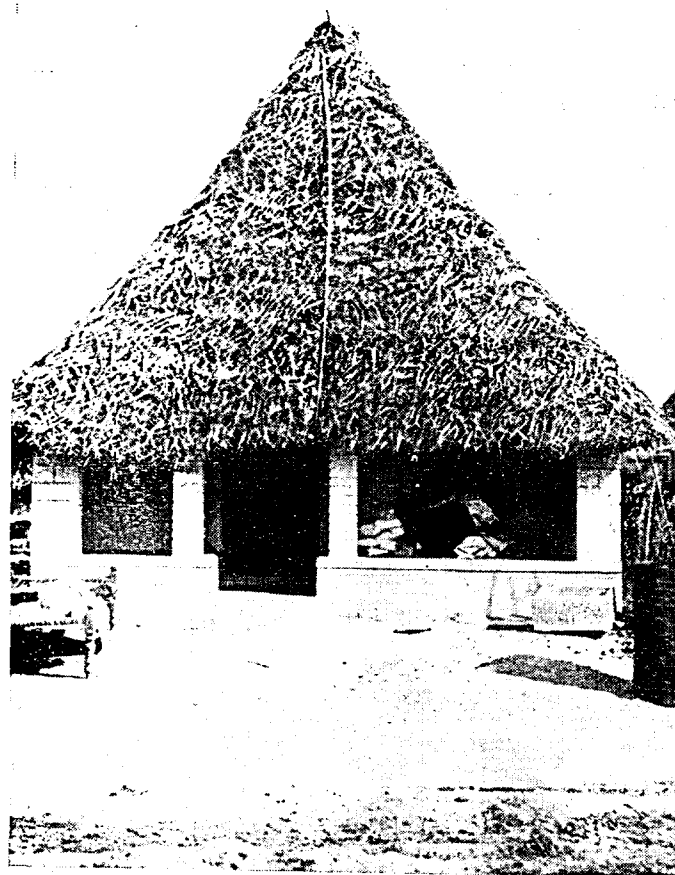
A completed dwelling.
