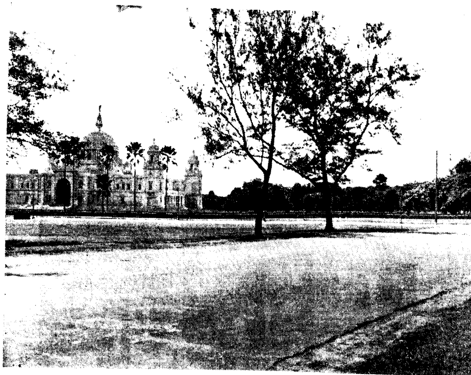
CASURINA AVENUE, Calcutta - 2" Grout as base course finished with 1" premix carpet as wearing course.
