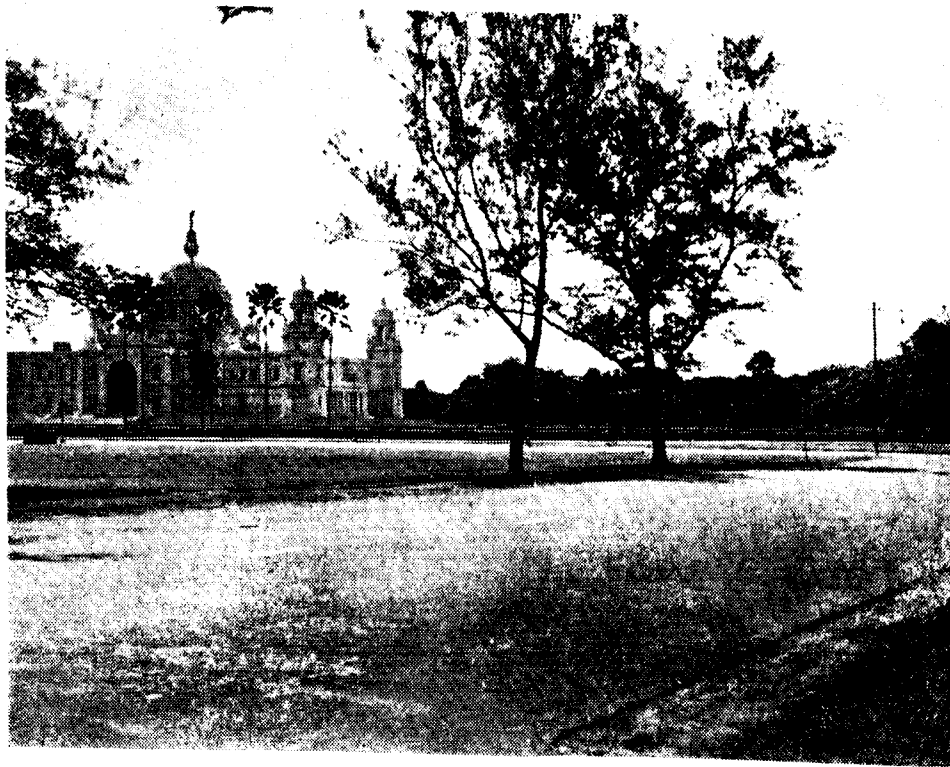
CASURINA AVENUE, Calcutta—2" Grout as base course finished with 1" premix carpet as wearing course.
