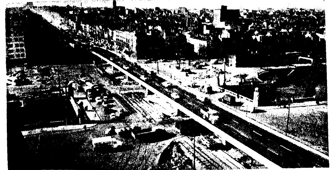
Viaduct at Place Saintelette, one of the express facilities completed in Brussels' Postwar program. (United Press Photo.)
