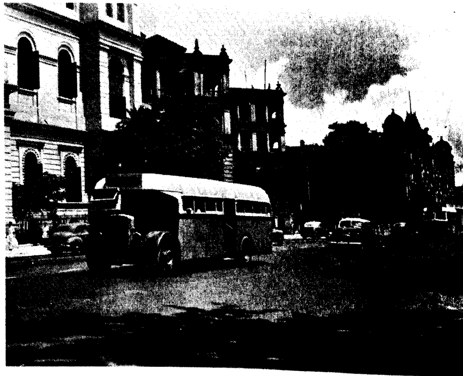
CHOWRINGHEE ROAD, Calcutta—3" Asphaltic concrete in two courses laid in 1953.
