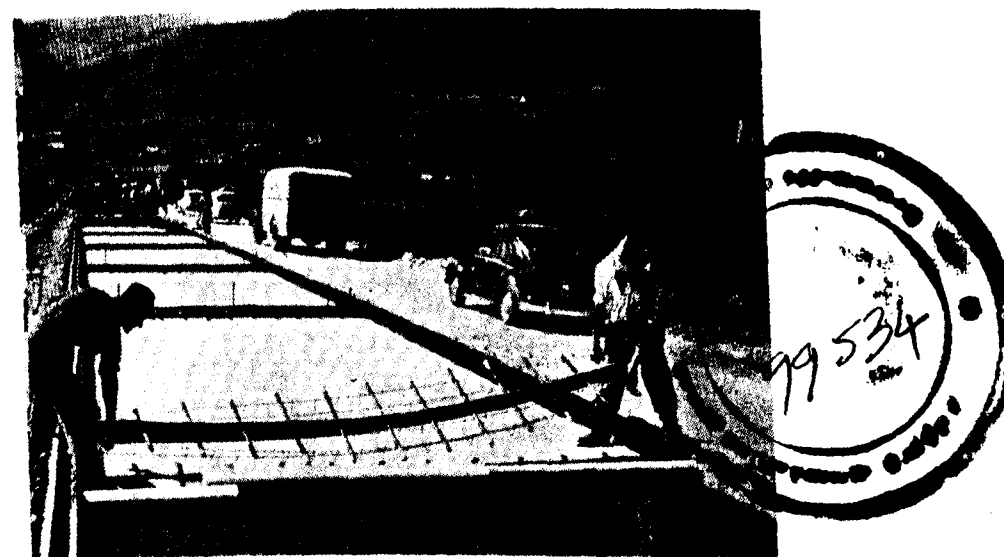
The Vienna-Trieste road under construction at Oberaich: dowel-bar assemblies are being placed in position.
