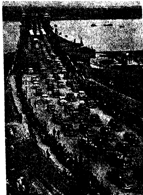
An endless stream of vehicles pass through the Yangtse bridge
