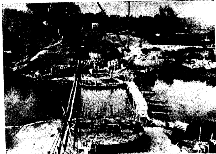
Photo 4. Islands for Wells Nos. 6 and 7: Bridge over piles between them
