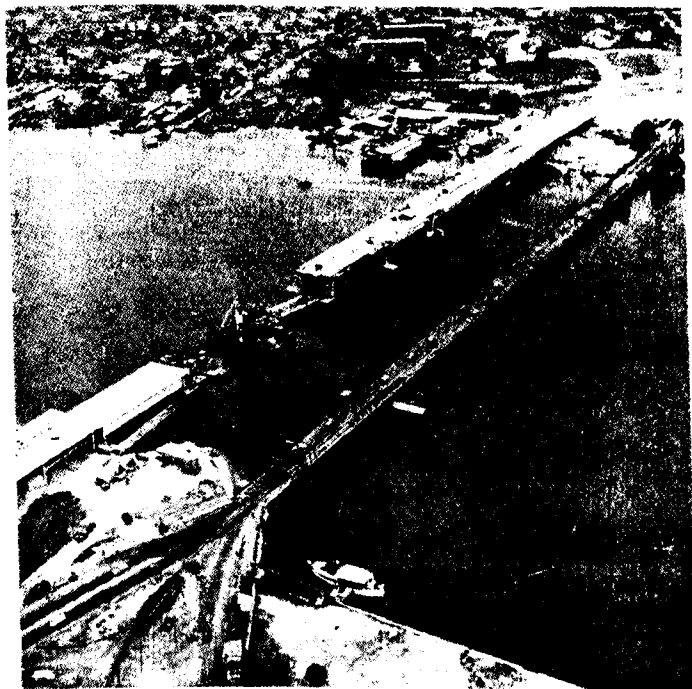
Aerial View of the Abidjan Bridge under construction with the Original Floating Bridge on the right (Enterprises Boussiron)
