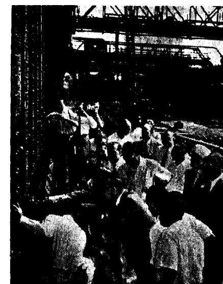
Lighting up of Tata Coke Oven Battery No. 3
