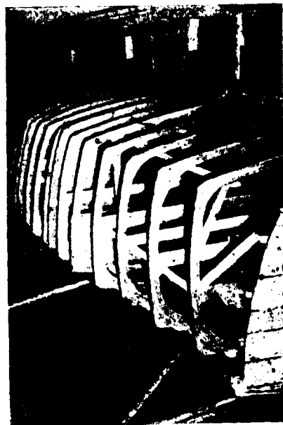
Keel Assembly showing laminated frames in position.
