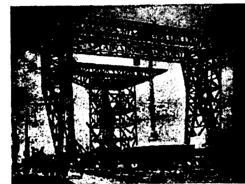
Goliath crane with its erecting platform at the rear. A load of 200 tons is suspended from the main hoist.
