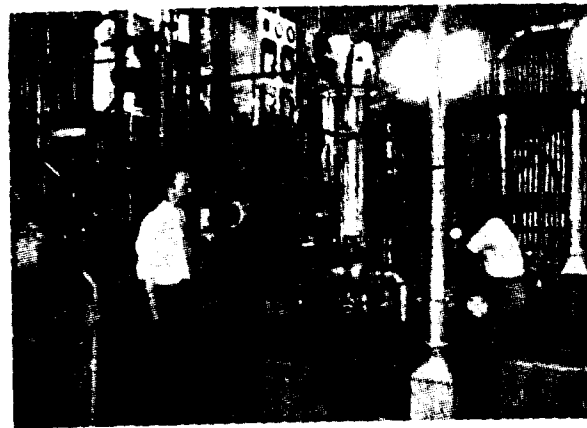
Fig. 3. Interior view of pilot plant showing cotton treating system.
