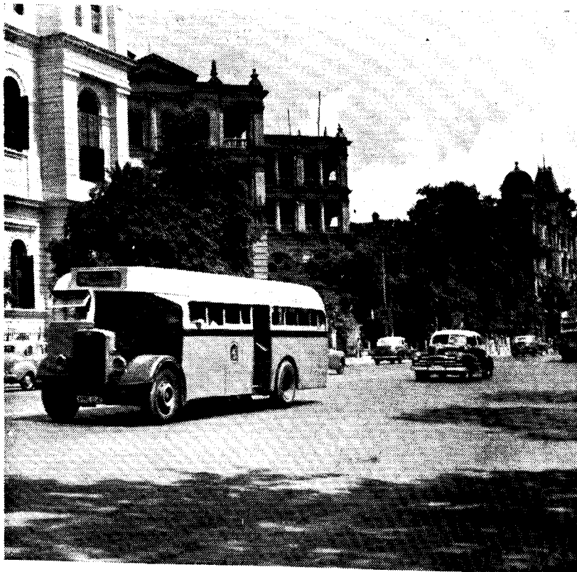
CHOWRINGHEE ROAD, Calcutta—3" Asphaltic concrete in two courses laid in 1953.
