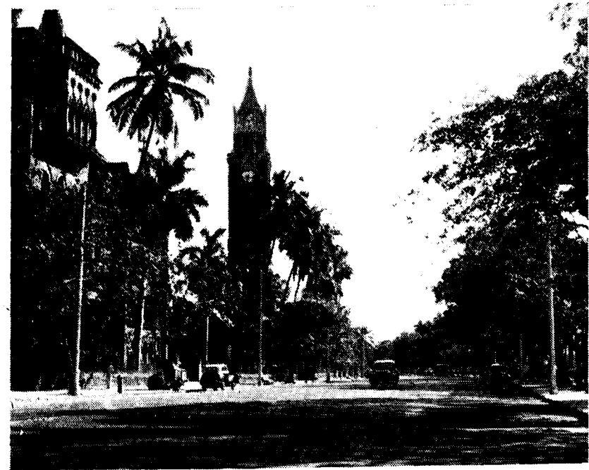
MAYO ROAD in Bombay—3/4" to 1" chipping carpet laid in 1956/57 using Burmah-Shell Bitumen.
