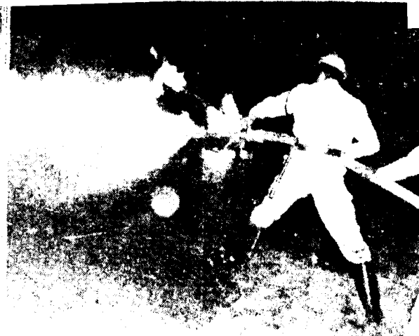
Fighting Oil Fire With Water projected through a fog nozzle
