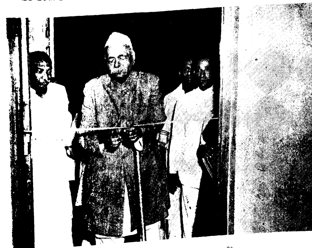
Maternity Centre building, constructed by the staff and inmates of the Govt. Care Camp, Melpakkam.
