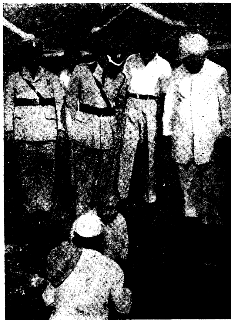
Shri M. M. Chudasama, I. P., Inspector-General, Bombay, laying the foundation stone of quarters for 68 constables in Surendranagar, Zalawad district police headquarters, Bombay State. The construction will cost Rs. 2,72,000.
