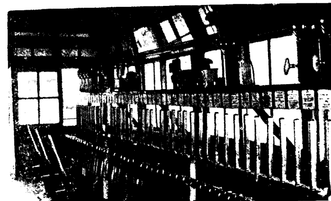
Interior of electro mechanical signal cabin in India. (Photo by the author)
