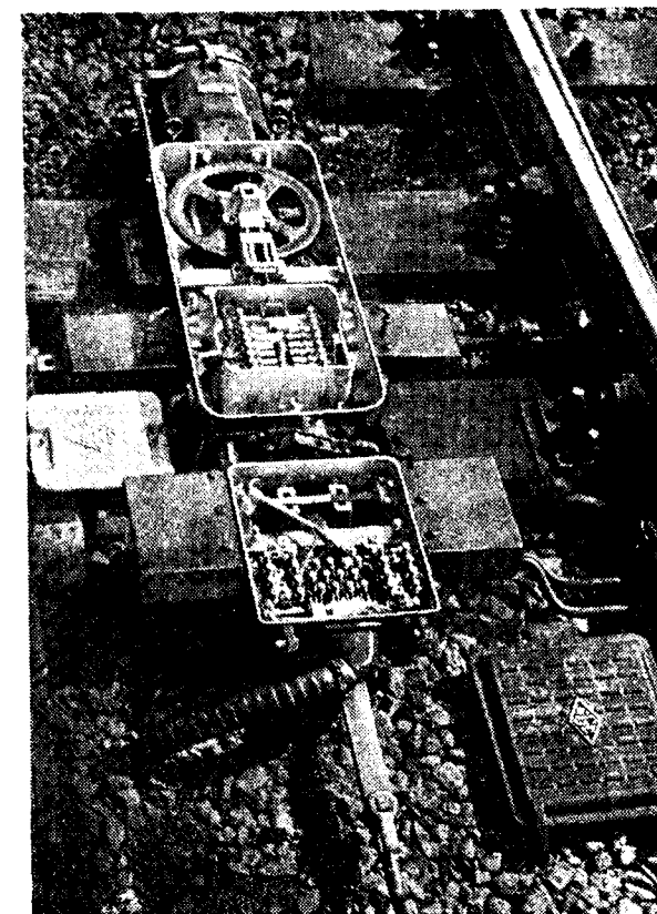
Installation of Type HB Combined Point Machine, 110 Volts D.C. showing contact box with double pole cut-off contacts.
